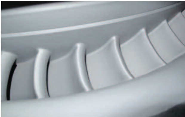
Figure 20 IP turbine blading at Waigaoqiao No 3 after 30 months' operation (Feng and Yu, 2012)
