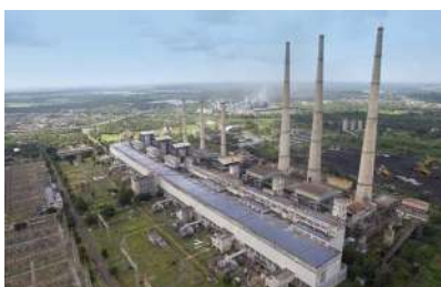
Kolaghat Thermal Power Station
