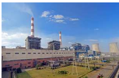
Sagardighi Thermal Power Plant
