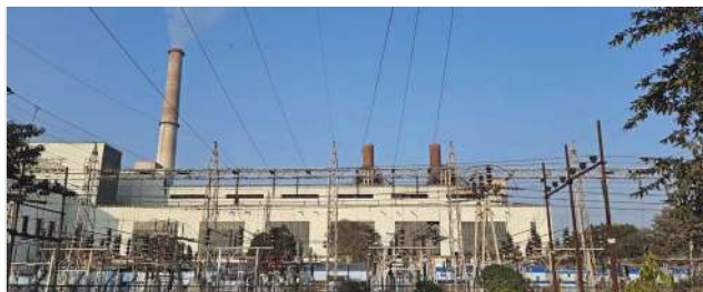
Bandel Thermal Power Station
