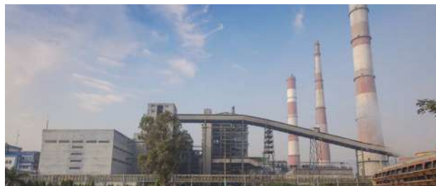
Bakreswar Thermal Power Plant
